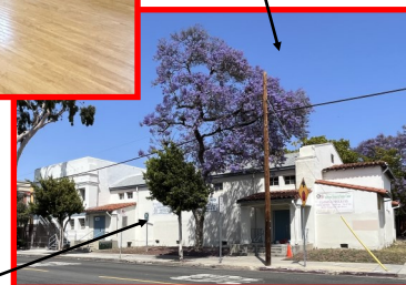
West side of the Building on Mesa Street
