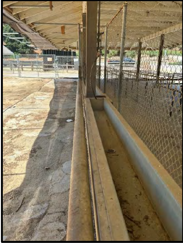
Figure 16 View of the troughs at the south side of the canopy.
