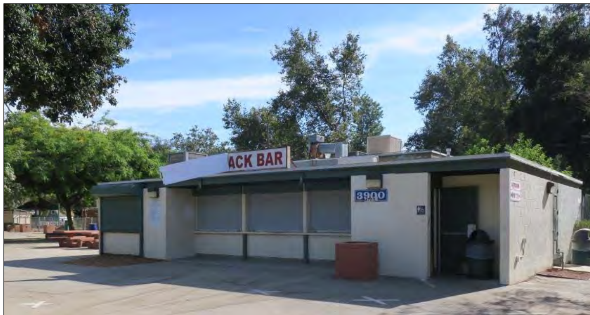
View northeast of the snack stand and restroom building (ARG, 2023).
