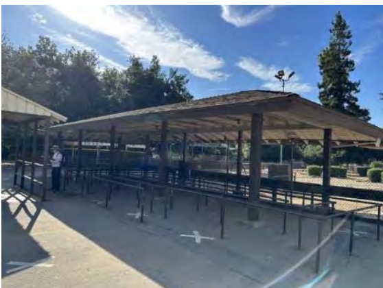
View looking southeast showing pergola and stanchions (ARG, 2023).
