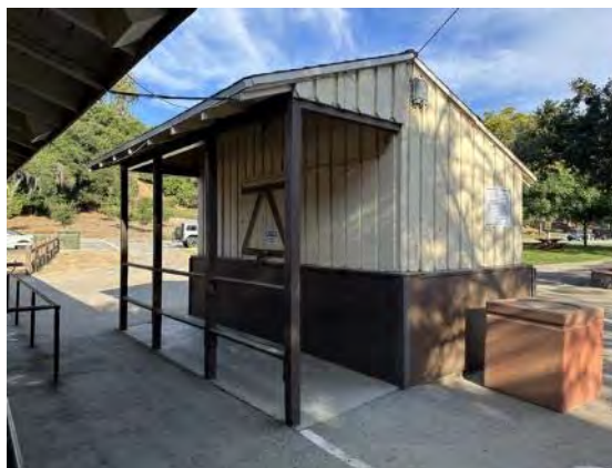
View looking northwest; note covered porch and ticket window (ARG, 2023).
