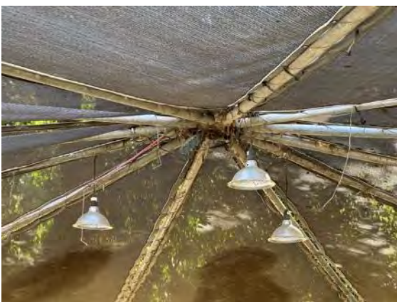
Detail at top of conical roof pipe framing and lights (ARG, 2023).
