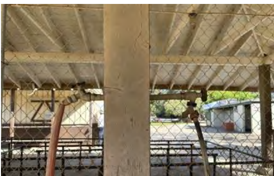
Detail at column with water spigots and hoses (ARG, 2023).
