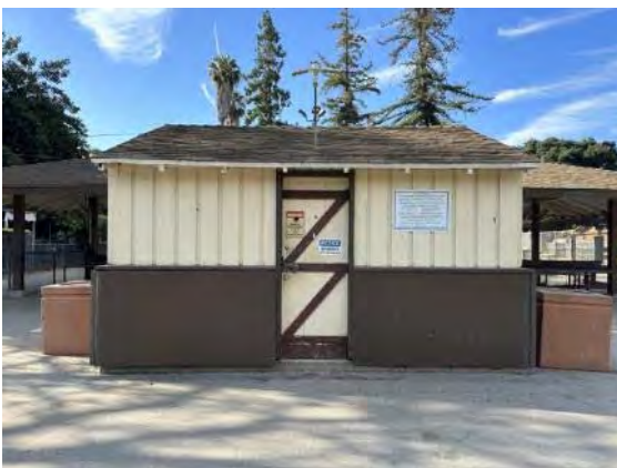
North façade of ticket booth (ARG, 2023).
