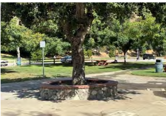
Circular planter to north of ticket booth (ARG, 2023).
