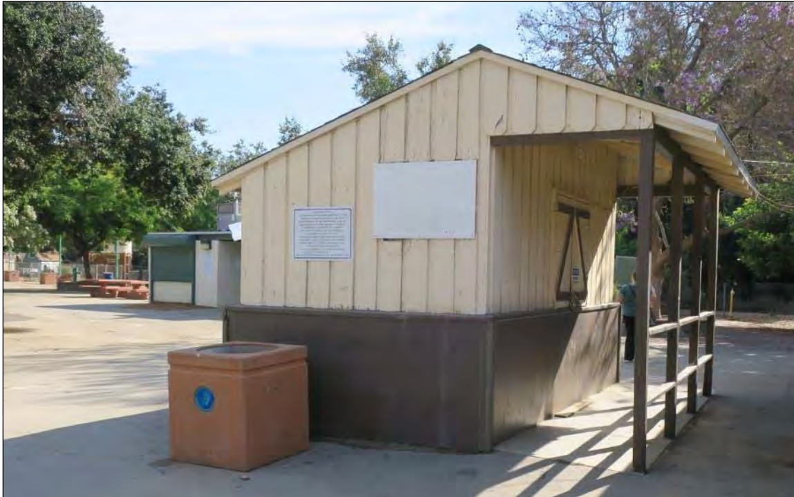
View west of the ticket booth (ARG, 2023).
