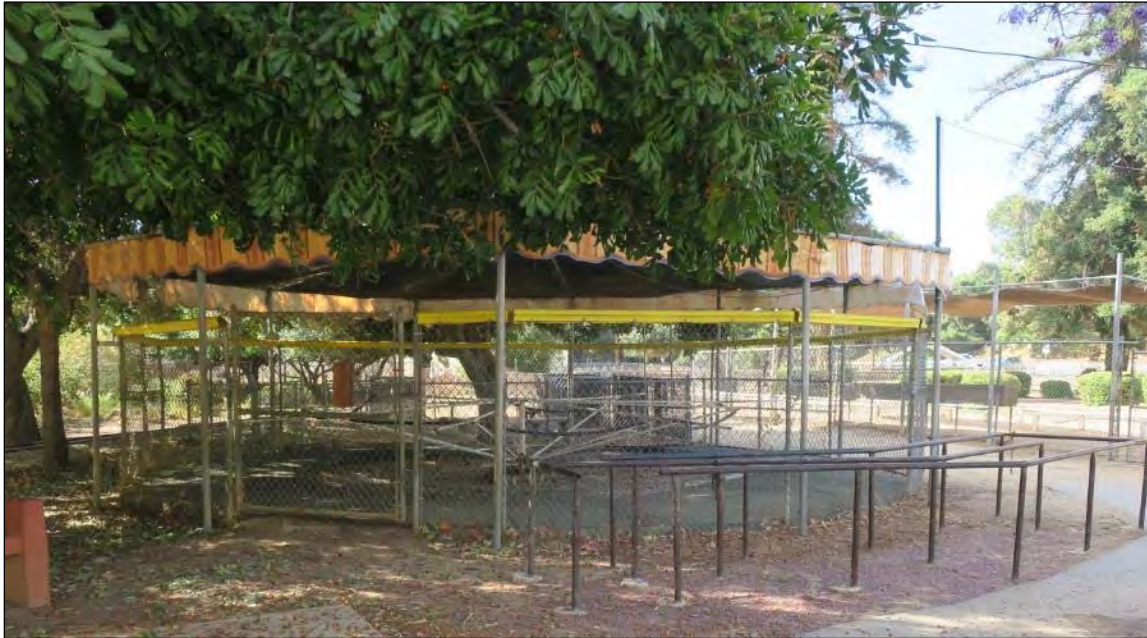
View south of the pony sweep (ARG, 2023).
