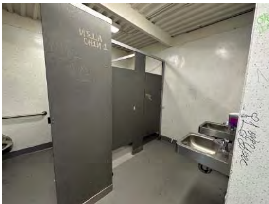
Interior view of women's restroom looking south (ARG, 2023).
