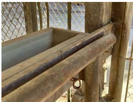
Detail at trough and tethering rail (ARG, 2023).
