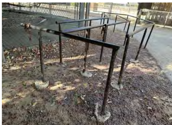
View of metal stanchions (ARG, 2023).
