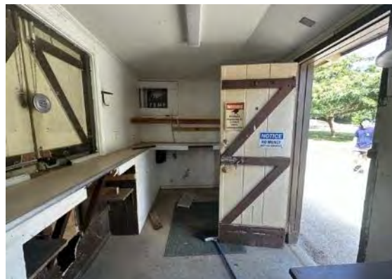
Interior view looking west (ARG, 2023).
