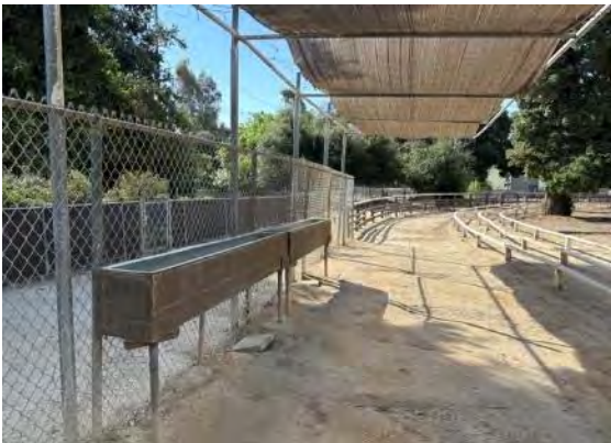
Shade structure and troughs at northeast corner of riding ring (ARG, 2023).
