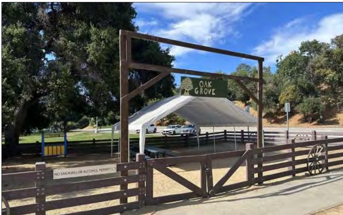
View southeast of the south “Oak Grove” birthday pavilion (ARG, 2023).
