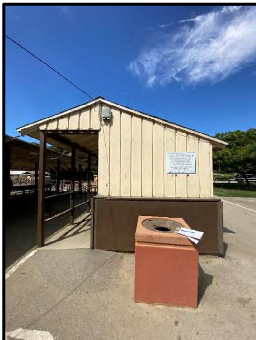
Figure 20 East elevation of the Ticket Booth showing the columns at the south.
