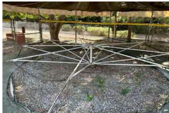
View of carousel at center (ARG, 2023).
