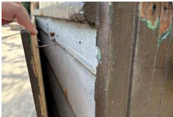
Detail near entrance; note horizontal siding beneath plywood wainscot (ARG, 2023).
