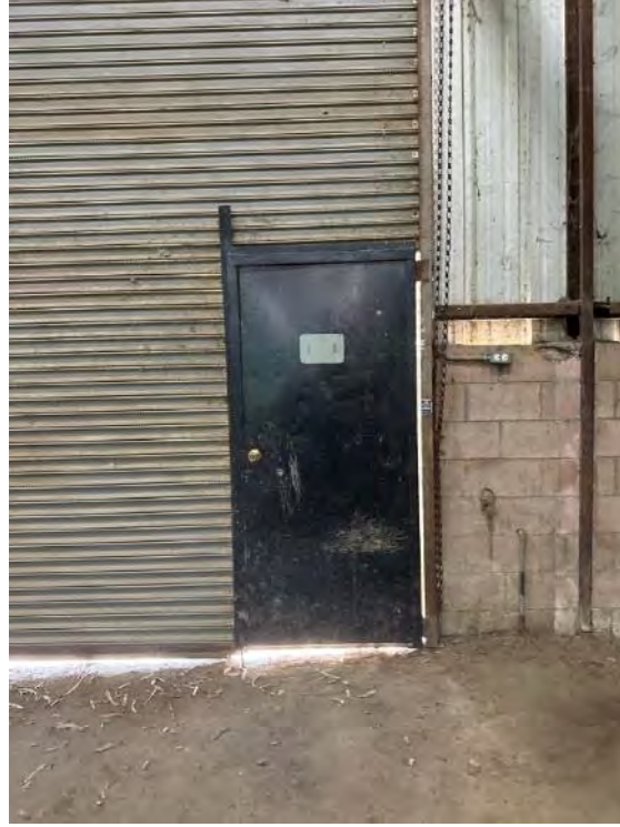
Detail at overhead door with pedestrian door inset (ARG, 2023).
