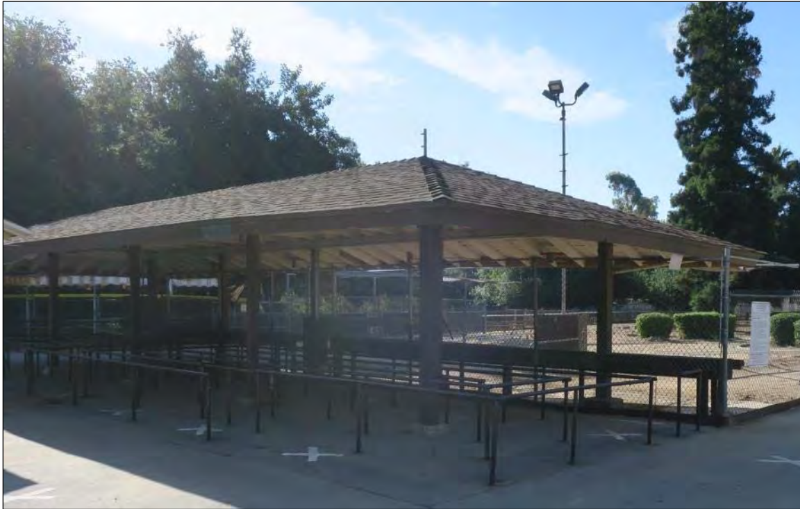
View southeast of the pergola (ARG, 2023).
