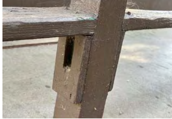
Detail at porch top rail; note wood bracket from previous railing (ARG, 2023).
