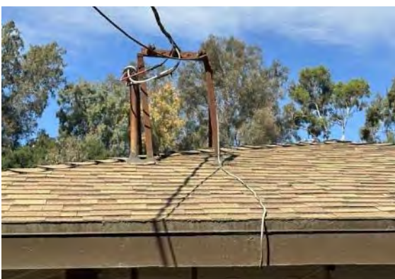
Detail at east side of roof showing cable support device (ARG, 2023).
