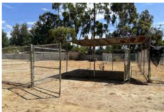
Shade structure and fencing at corrals (ARG, 2023).
