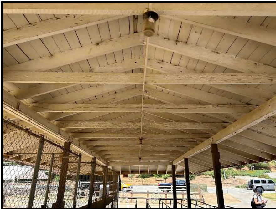
Figure 15 View of the Pergola roof collar ties, rafters, and beams.
