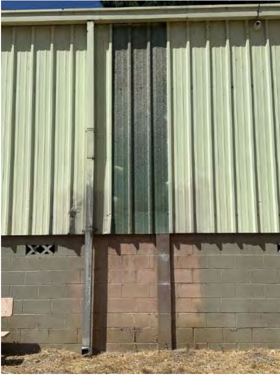
Detail at east exterior wall; note corrugated polycarbonate "window" panel (ARG, 2023).
