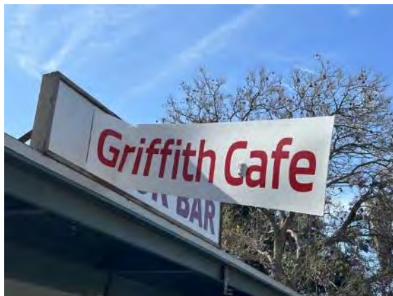
Loose temporary sign over existing illuminated sign (ARG, 2023).
