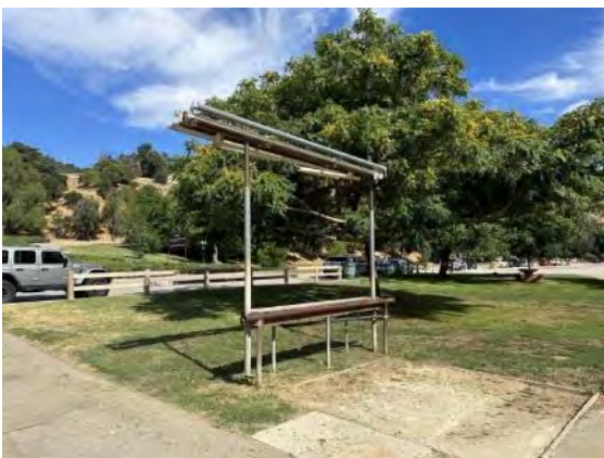
View of freestanding shade structure (ARG, 2023).
