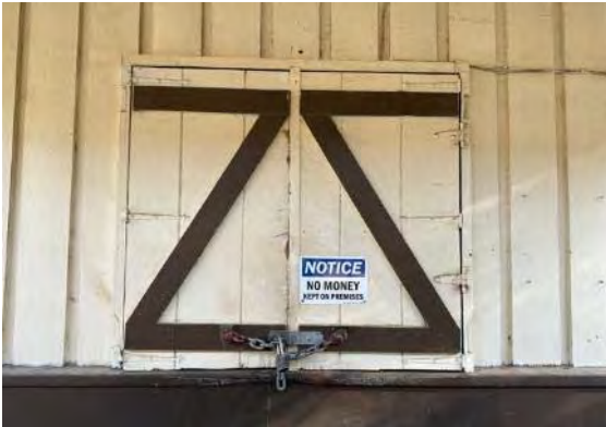
View of ticket window exterior shutters (ARG, 2023).
