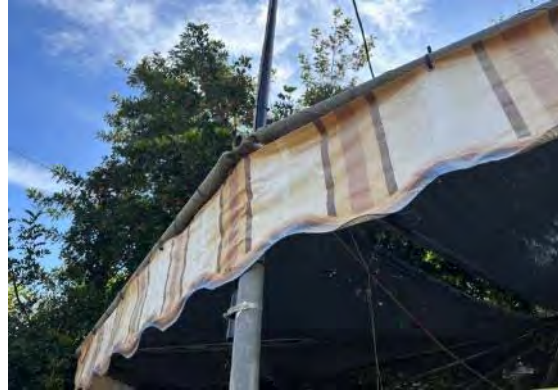
Detail at valance; note faded colors (ARG, 2023).
