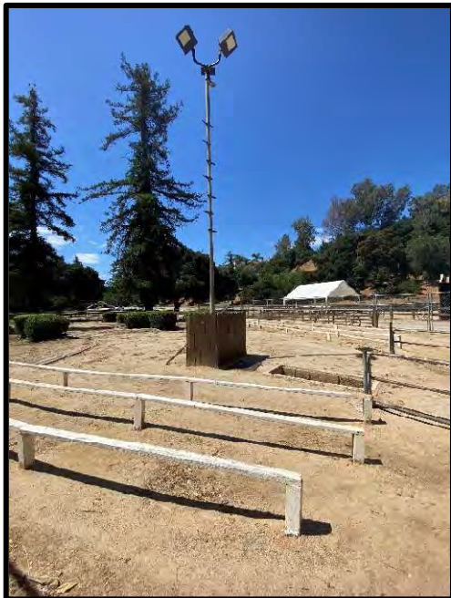
Figure 31 View of the light post.
