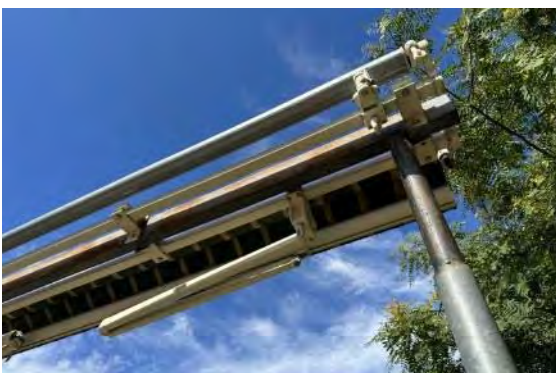
Detail of retractable awnings (ARG, 2023).
