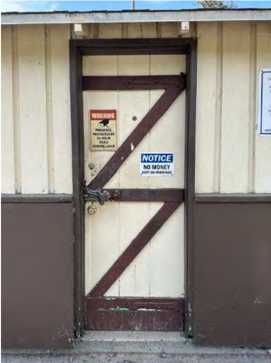
View of door exterior; note added base trim (ARG, 2023).
