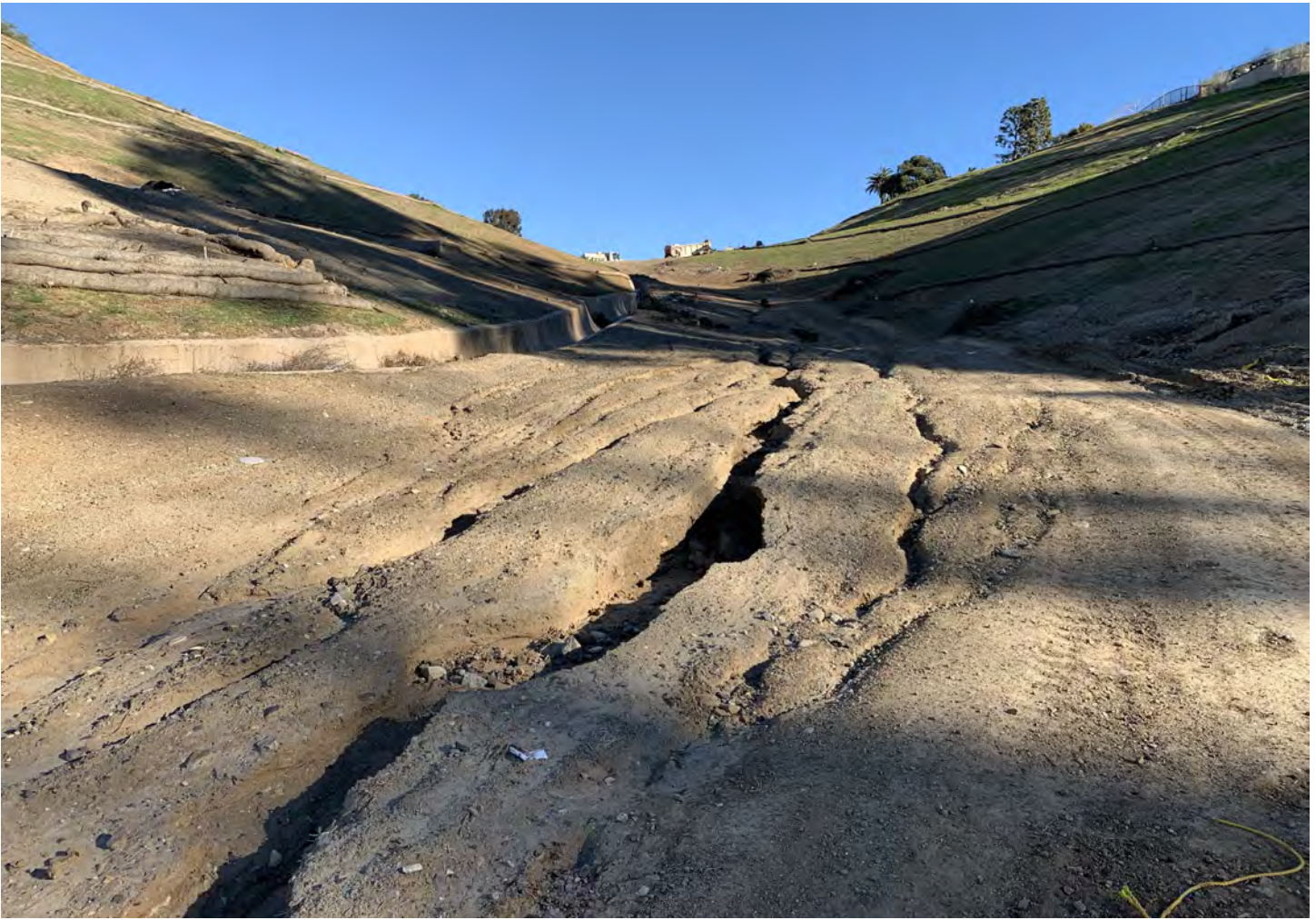
Photo 3 (above): Looking north into the canyon. Heavy rains resulted in severe erosion gullies that made the roadway unsafe for construction vehicles to enter the canyon.
