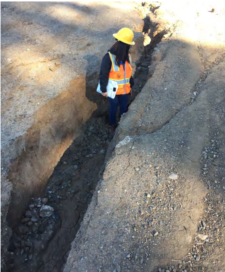
Photo 3 (above): Looking north into the canyon. Heavy rains resulted in severe erosion gullies that made the roadway unsafe for construction vehicles to enter the canyon.
