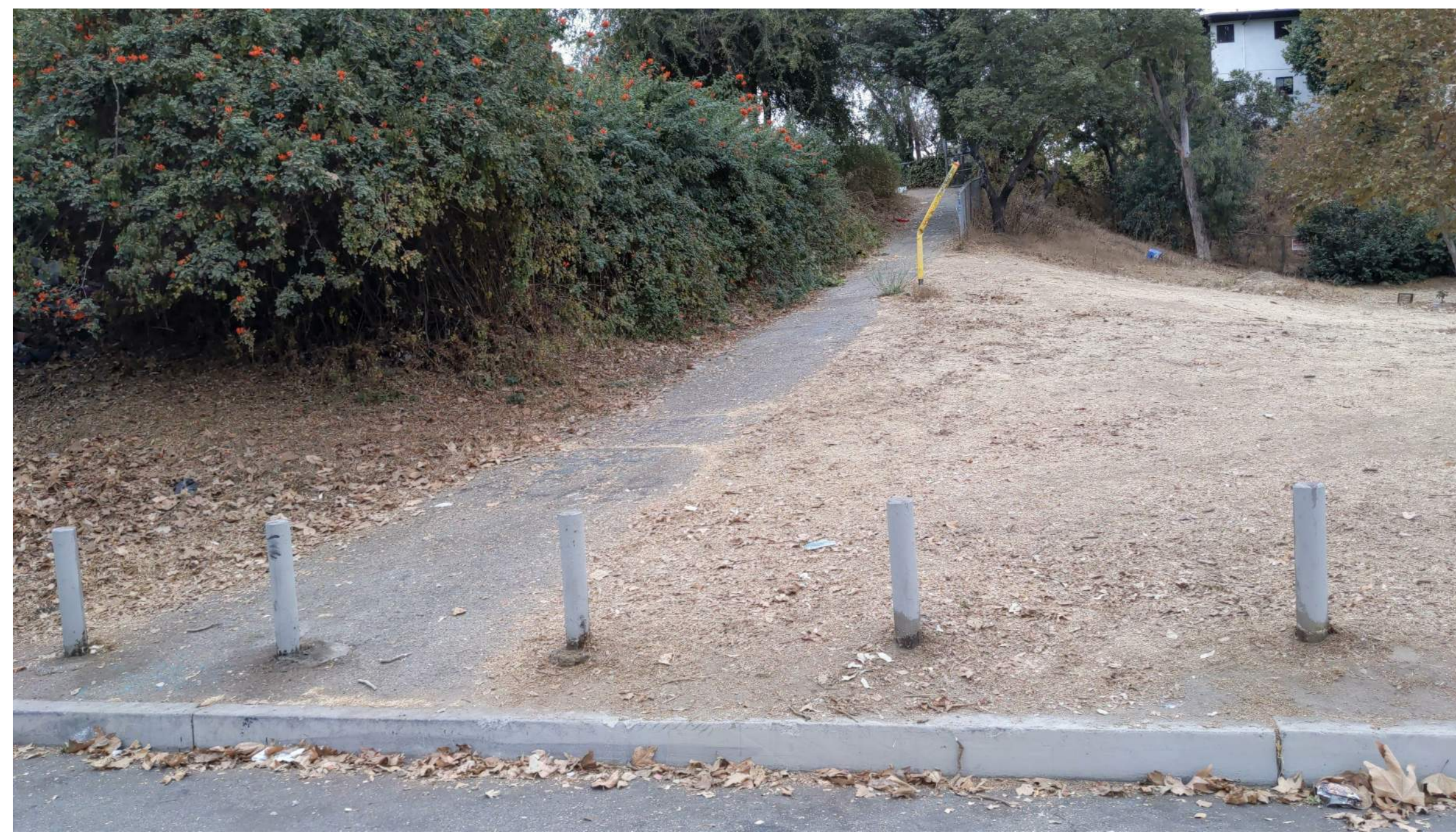
WALKWAY ENTRY FROM AVENUE 60
