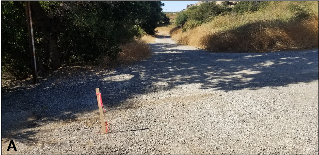
Photo A, facing south, showing survey markers for proposed trenching of the pipeline.
