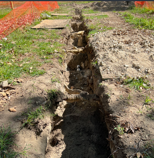
Tunneling under California sycamore roots at Arroyo Seco Ave 60 Park.
